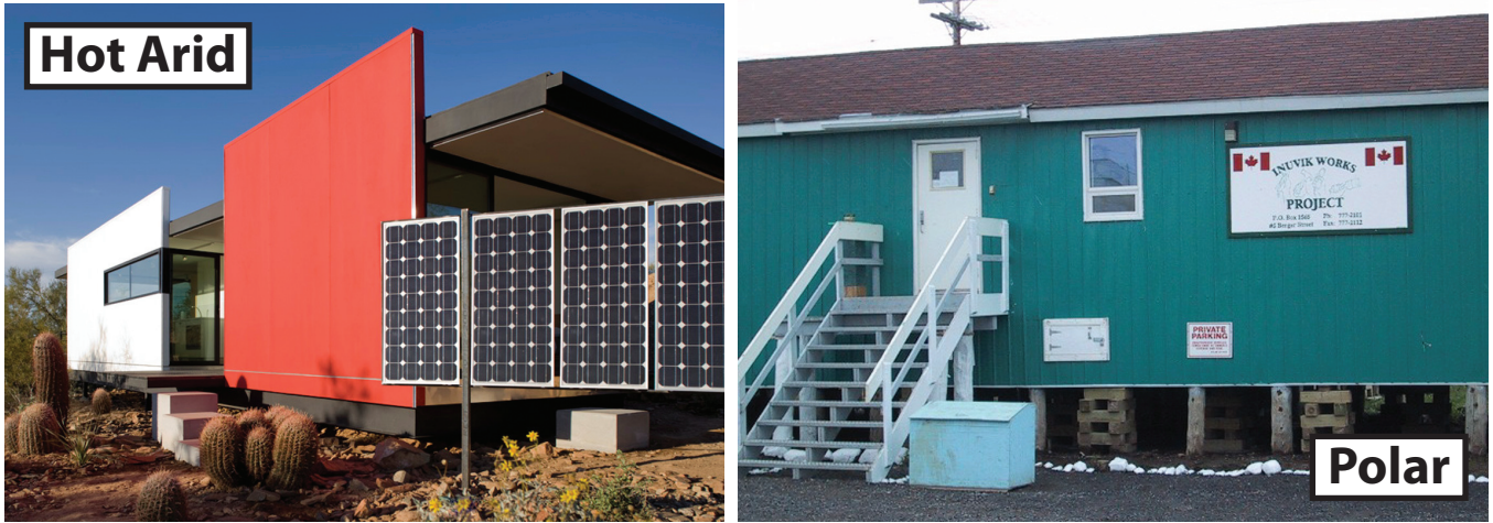
Figure 8 – Buildings adapted to cope with extreme climates
