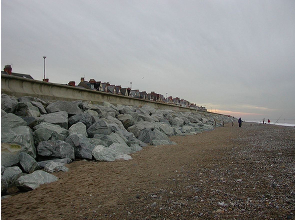
Figure 5 – Photograph of Coastal Defences
